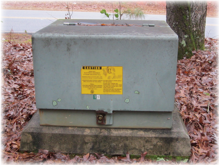
Padmount Transformer, Power Box, or Cabinet
