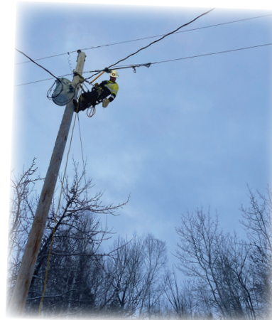
CLP lineman repairing damaged wire.
